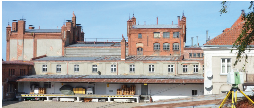
Fig. 1. Laser scanner seen against the oldest part of the brewery – a view on the southern façade on the court side
