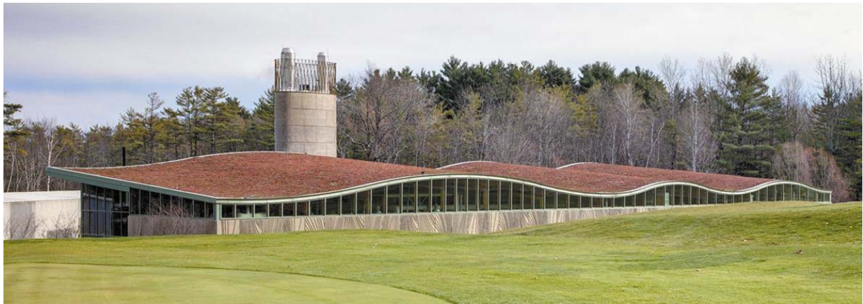
Fig. 10. The roof of the incineration building at the Hotchkiss School campus, Salisbury, USA (©O&G Industries, source: https://www.ogind.com/sites/default/files/styles/flexslider_full/public/portfolio/h-biomass-primary.jpg?itok=6_Zy7ZIJ )
