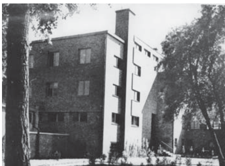
Fig. 11. The Post Office building in Ciechocinek, the side elevation [Architektura i Budownictwo 1937, 3, 70–73]
