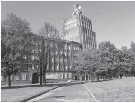
Fig. 7. The Post Office building in Wrocław, a general view (photo by Z. Borcz)
