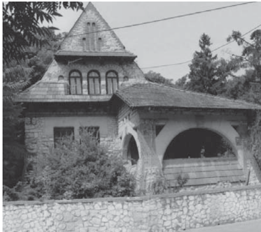
Fig. 5. The kindergarten building in Nałęczów, designed by J. Witkiewicz-Koszczyz (photo by Z. Borcz)
