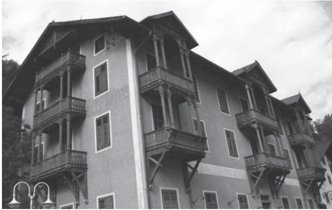
Rys. 17. Wykusze w alpejskim kurorcie Sand in Taufers, Włochy (fot. I. Niedźwiecka-Filipiak) Fig. 17. Bays of buildings in the Alps health resort Sand in Taufers, Italy (photo I. Niedźwiecka-Filipiak)
