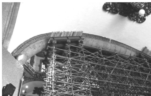
Fig. 20. Temporary protection of arch vault (photo by author)
