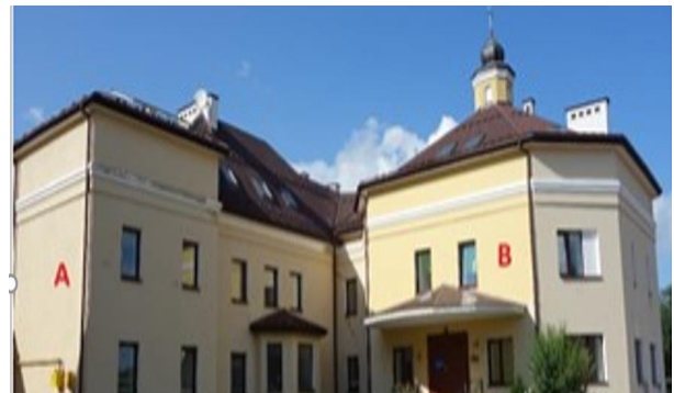
Fig. 1. Buildings' layout: A – the northern part; B – the southern part of the multi-storey building at Port Harcourt (photo by the author)
