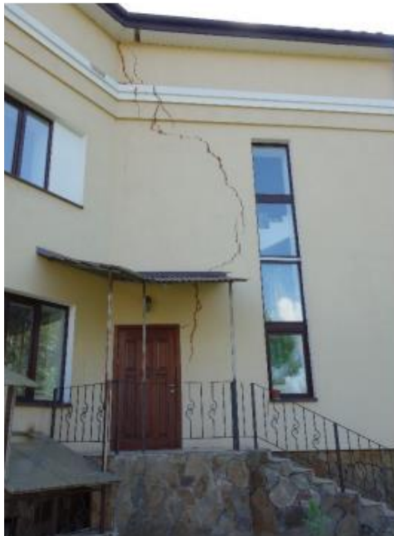
Fig. 2. Scratches of the external bearing wall of the linking part between the northern and southern part of the building (photo by the author)
