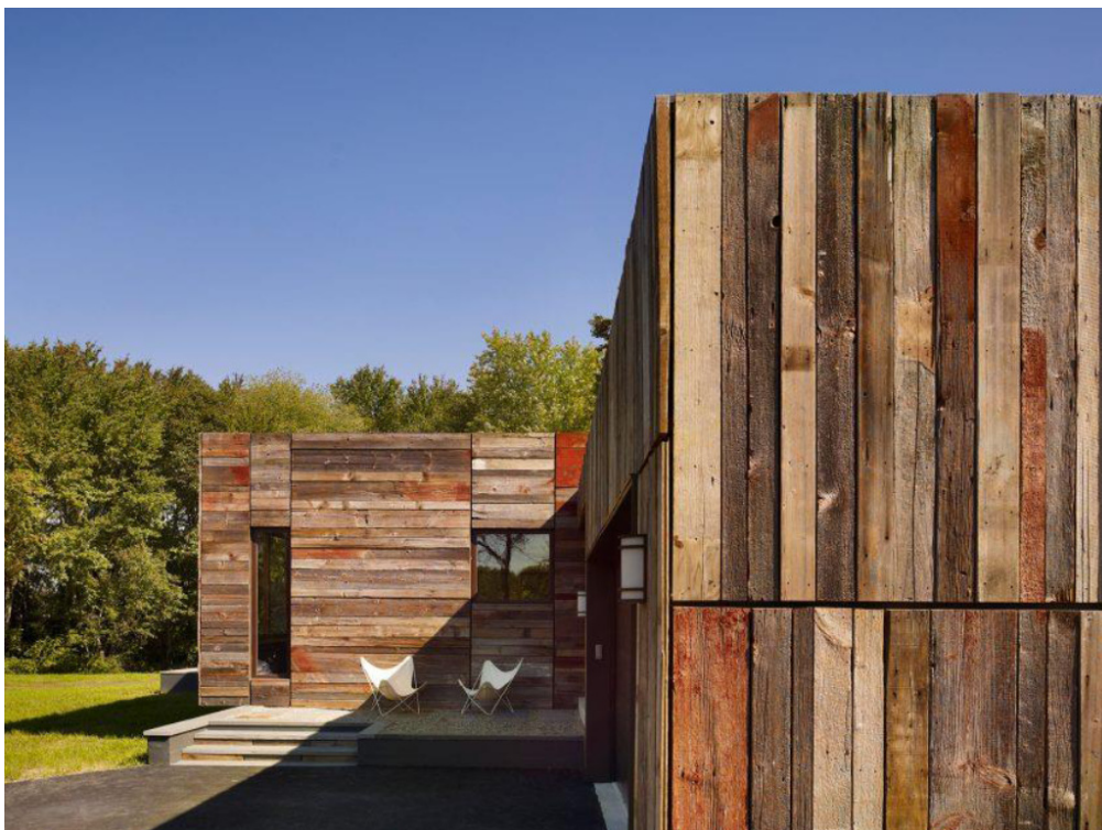
Fig. 1. Old barn wooden covering
