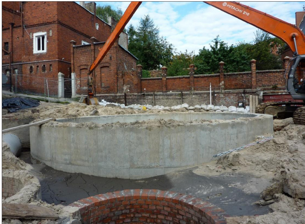
Fig. 9. Construction works on sinking the well in Bydgoszcz (the author's photo)
