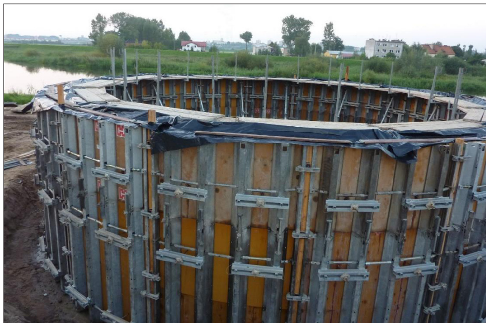
Fig. 10. Construction works on sinking the well in Konin (the author's photo)
