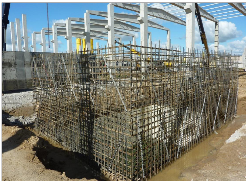
Fig. 12. Construction works on sinking the well in Sobota (the author's photo)
