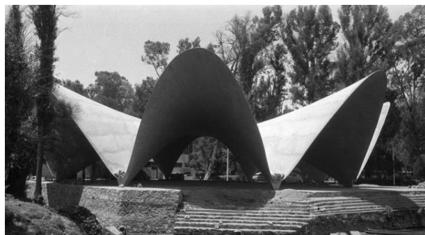
Fig. 6. Los Manantiales, Mexico City, 1958 – restaurant designed by Félix Candela
