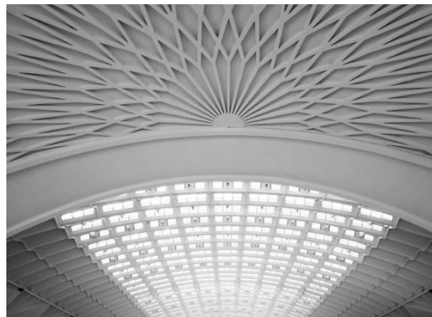
Fig. 2. Palazzo di Torino Esposizioni (Saloni C), Turin, 1948 – art exhibition hall designed by Pier Luigi Nervi (photo by M. Carrieri)
