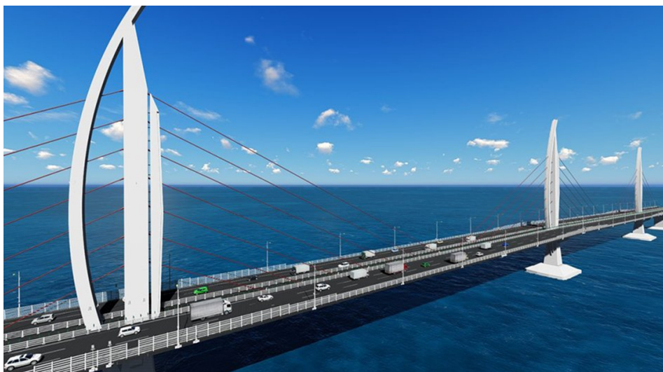
Fig. 1. 3D-model of a part of the Hong Kong-Zhuhai-Macau bridge ( https://damassets.autodesk.net/content/dam/autodesk/drafter/4358/cropped-1534866310.jpg )
