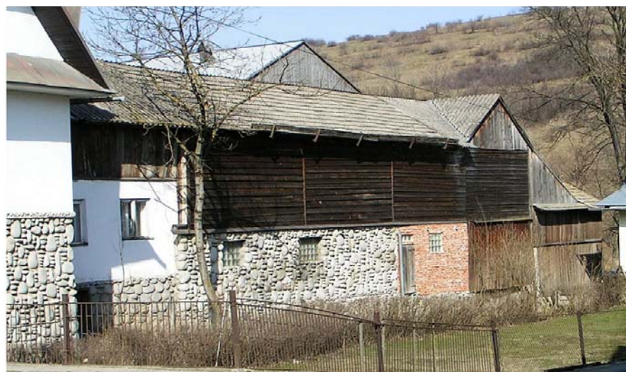
Fig. 9. The wall of a farm building in Trybsz with a high knee wall and various construction materials used (photo by P. Herbut)
