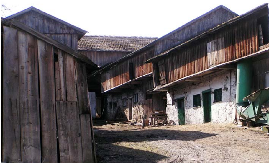
Fig. 7. Farmyard in the middle part of Trybsz. Visible overhanging attics over farm buildings (photo by P. Herbut)
