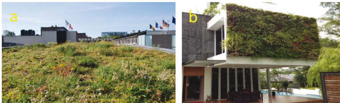
Fig. 4. Biodiverse green roof: a – an office building, the Netherlands; b – a living wall of a private residence, the Netherlands (Sempergreen BV, 2017)
