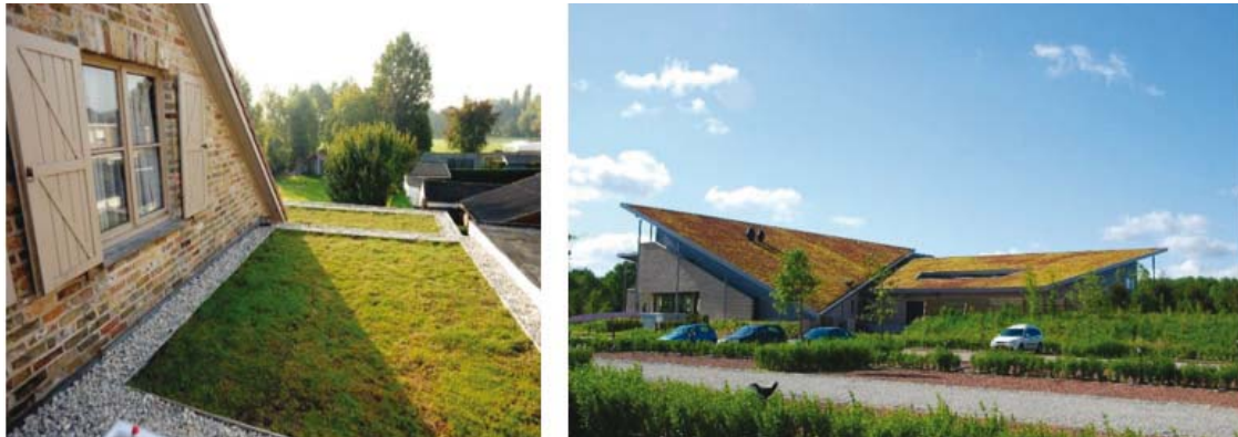
Fig. 3. Extensive roof, the Netherlands (Sempergreen BV, 2017)
