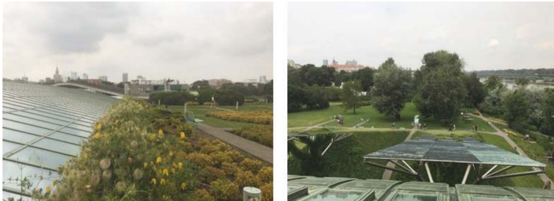
Fig. 1. Warsaw University Library roof garden (photo by M.D. Vaverková, 2017)
