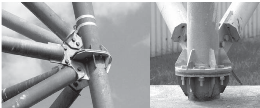
Fig. 3. Photographs of typical tower's joints
