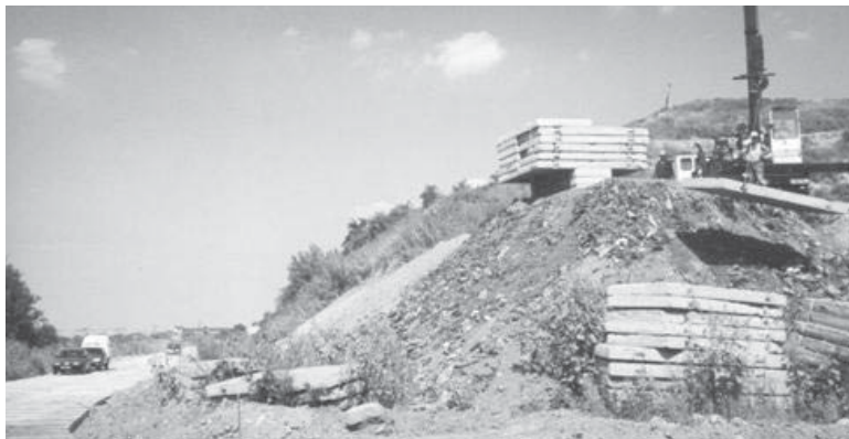
Fig. 3. Trial loading of the experimental embankment constructed on Radiowo landfill [Koda 2011]
