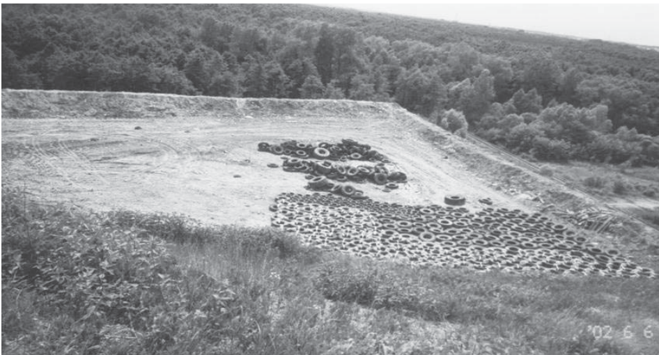
Fig. 7. Construction of the used tires mattresses layers on Radiowo landfill [Koda 2012]
