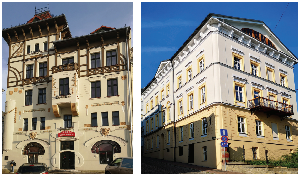
Fig. 5. House at Wojska Polskiego Square (on the left), tenement house at 2 Waryńskiego Street (on the right) in Bielsko-Biała after renovation
