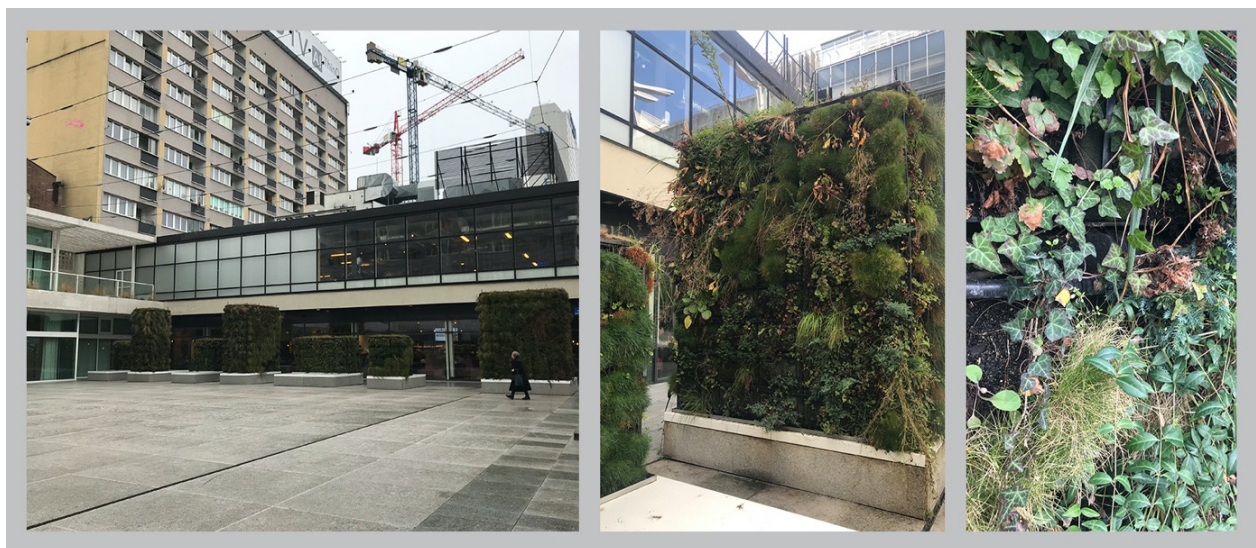
Fig. 4. Surface greenery systems in the square in front of the Warsaw Zodiac Pavilion of Architecture (photo by A. Nowak)
