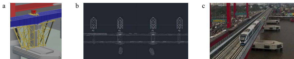
Fig. 18. Palembang LRT cross Musi river, Indonesia: a – modelling pier studies, b – plan view of pier foundation; c – LRT bridge after construction
