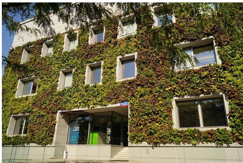
Fig. 2. Green wall on Foundation for Polish Science building in Warsaw (source: https://www.fajneogrody.pl/2015/08/zielona-sciana-mokotowie.html , accessed 05.09.2018)
